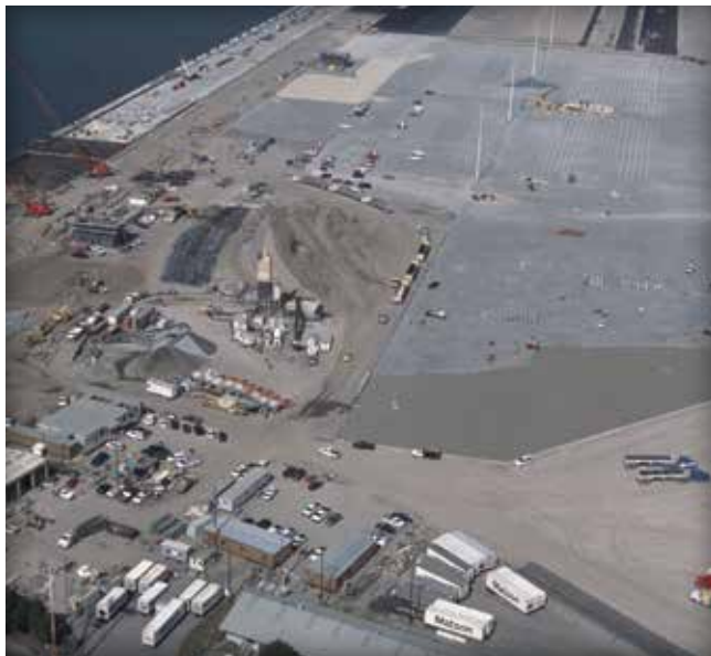
Figure 14. The Port of Oakland, California, is the largest mechanically installed project in the western hemisphere at 4.7 million sf (470,000 m 2 ).
